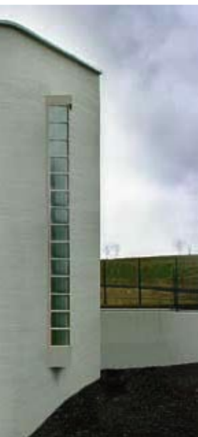
Ljósifoss station after renovation 2000.
