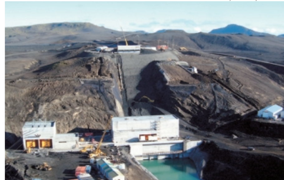
Vatnsfell Station in September 2001
